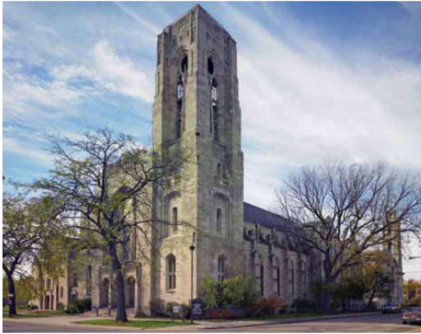
AltusWorks performed an extensive Facilities Analysis of the First Presbyterian Church complex in Chicago, IL.
